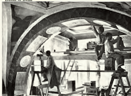
70. MASONS AND PAINTERS AT WORK Chapingo
