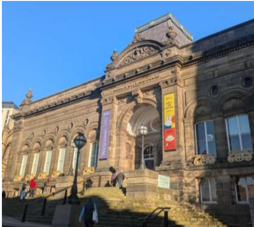
Figura 13. Fachada del Leeds City Museum. Fuente: https://www.facebook.com/photo/?fbid=1263650699101399&set=pb.100063694417321.-2207520000
